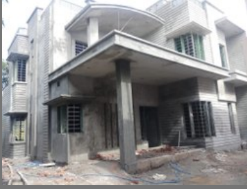
Hotel Building Construction Service
