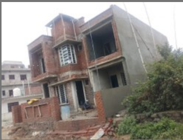
Office Building Construction Services
