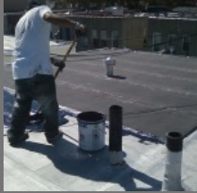
Structural Water Proof Service
