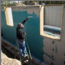
Cement & Epoxy Grouting Service
