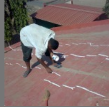
Expansion Joint Treatments Service
