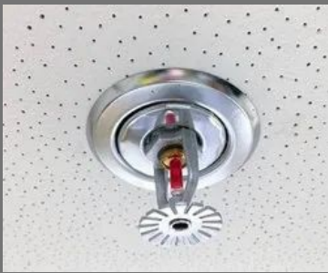
Fire Sprinkler Installation Services
