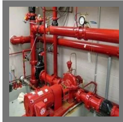
Fire Hydrant AMC Service
