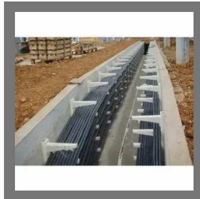
Electric Cable Laying And Installation
