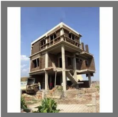
Civil Work Services
