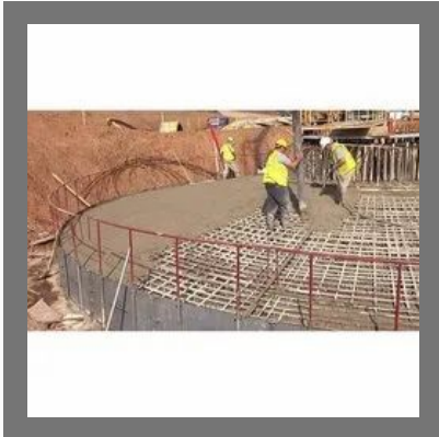
Civil Construction Contractors
