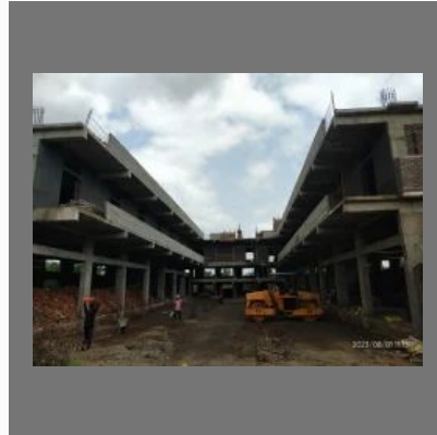
School Building Construction
