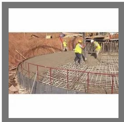
Civil Construction Contractors
