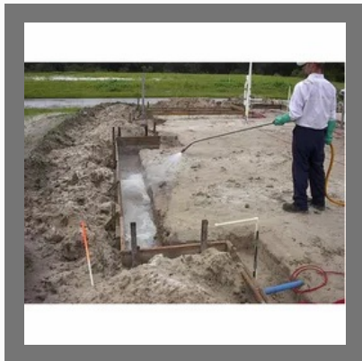
Anti Termite Treatment For Soil
