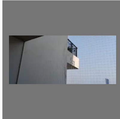
Balcony Netting in Gurgaon
