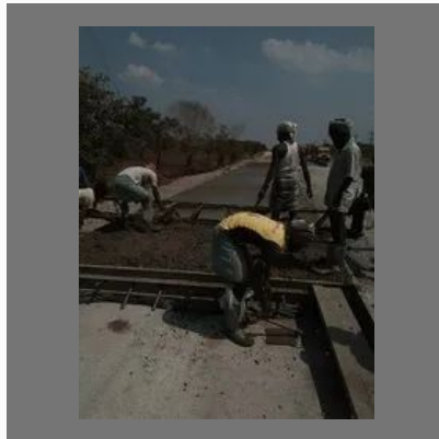
Vdf and truss screed flooring service
