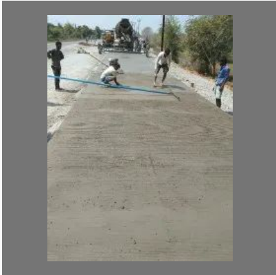
Vaccum Dewatering Flooring And Broom Finish Road Work Concrete
