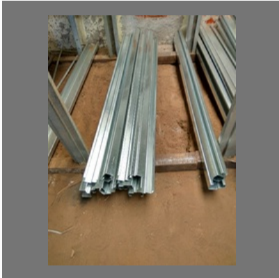
Gi Frame Fabrication Work
