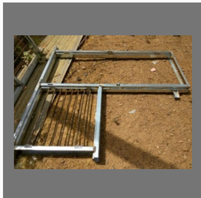
Double Doors Fabrication Work
