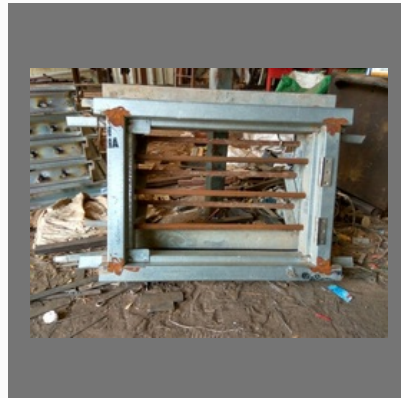
Windows Fabrication Work
