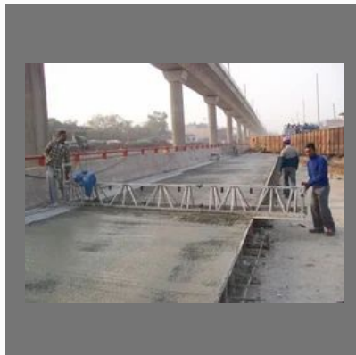
Concrete Truss Paver
