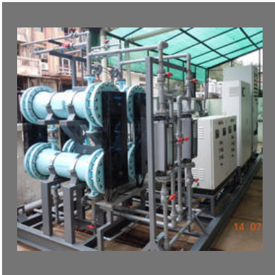
Electrochlorination Plant
