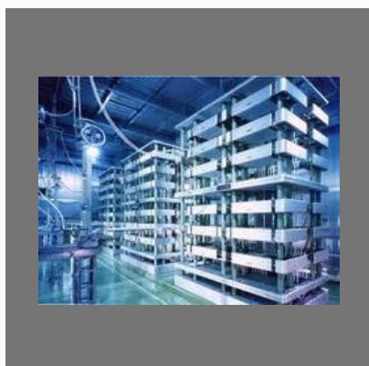
Hvdc Simulation and Fault Analysis of HVDC
