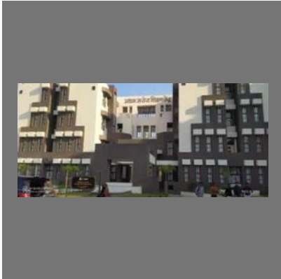
School Building Construction Service
