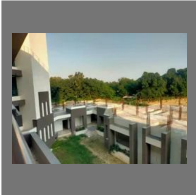
School Building Construction
