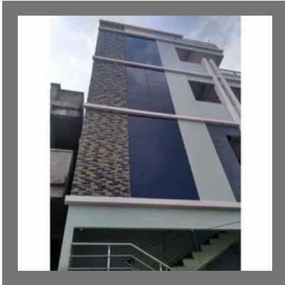
ACP Structural Glazing
