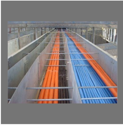
Electrical & Instrumentation Fabrication, Erection And Commissioning Services
