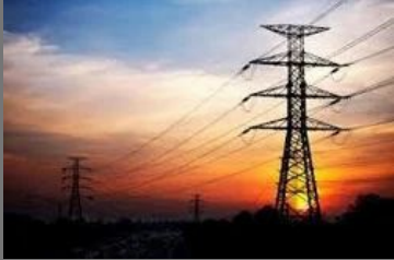
Power Distribution IT Solution
