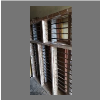
Window With Steel Pipe
