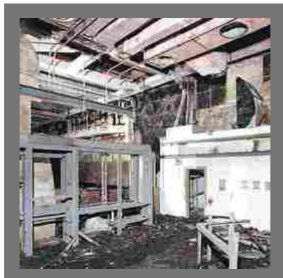
AC Plant Scrap
