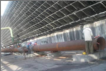
Piping equipment Thermal Insulation painting
