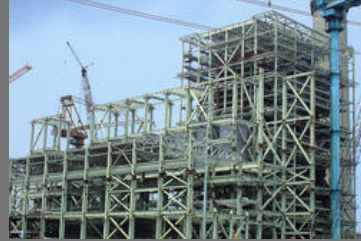
Building Steel Structure
