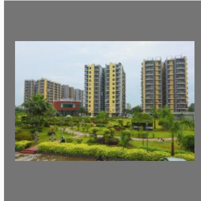
Maxxon Trishla City Ready To Move 2bhk 3bhk Flats
