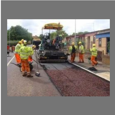
Road construction service
