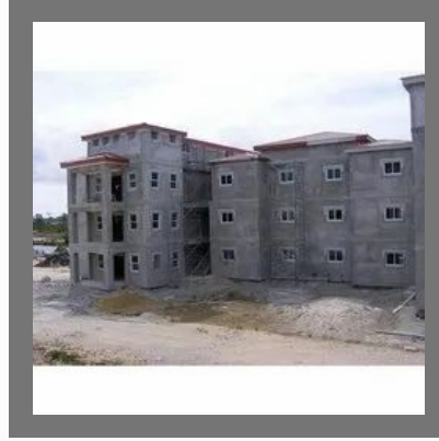
Construction Services For School Building
