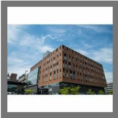
Construction Services For Hospital Building
